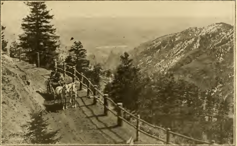
ON BEAR CREEK CANYON ROAD
